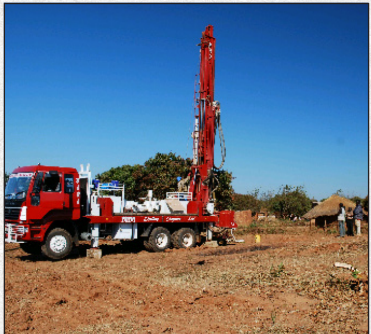
Deep Well Drilling Rig: 50-75 Meter Depth
